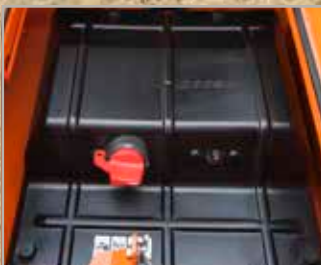
Battery cut-off switch
